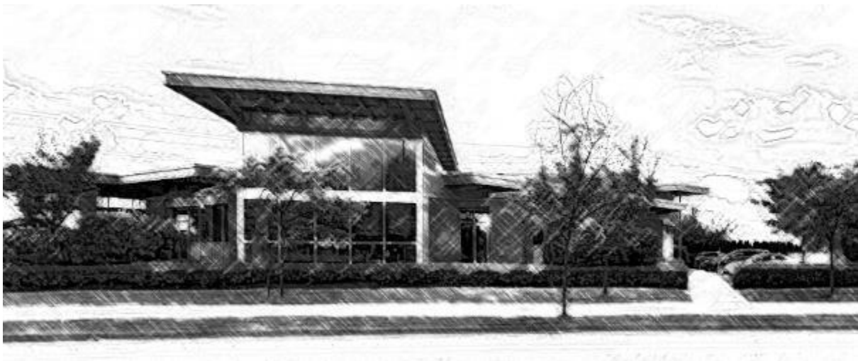
Figure 25: Building showing architectural detail
